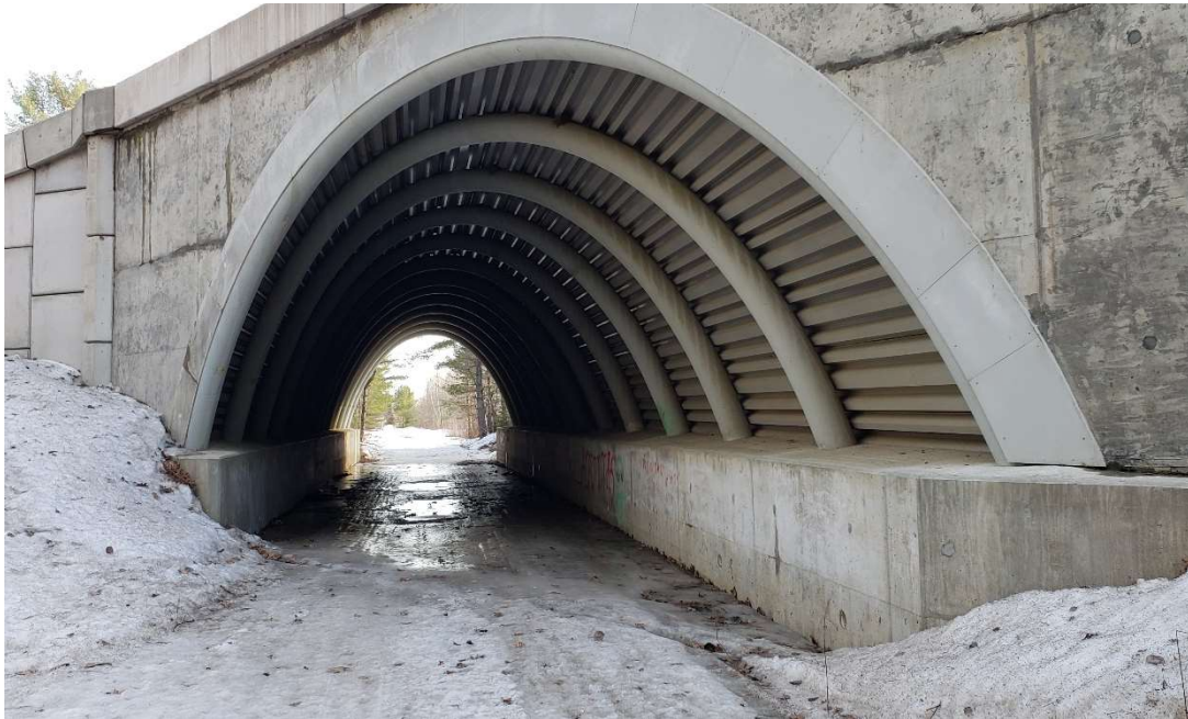
Figure 4-1. B&A Overhead Bridge in Lagrange, Maine, USA (consists of 13 CFRTs)
