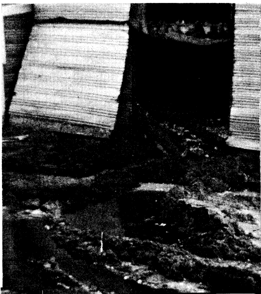
Chicken slurry oozes from Eggs Unlimited building. Slurry had built up over a period of years before forcing its way out.
