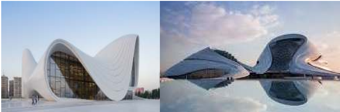
Gambar 1.3 Desain Neo-futuristik: Heydar Aliyev Cultural Centre, Zaha Hadid (kiri) Harbin Opera House, MAD Architect (kanan)
