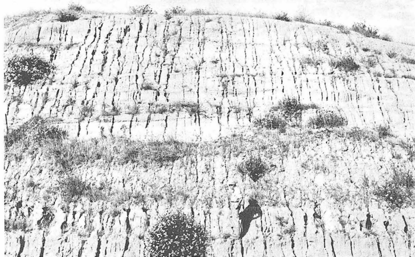
FIGURE 8. Roadcut exposure of poorly consolidated arkosic sandstone and pebble conglomerate near Temecula. This valley fill is late Pleistocene in age, and is a part of the Pauba formation of Mann (1951).
