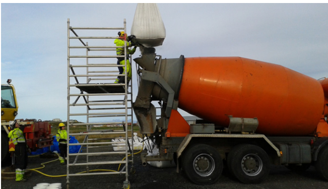
Fig. 10. Batching of high performance concrete inside a truck mixer.
