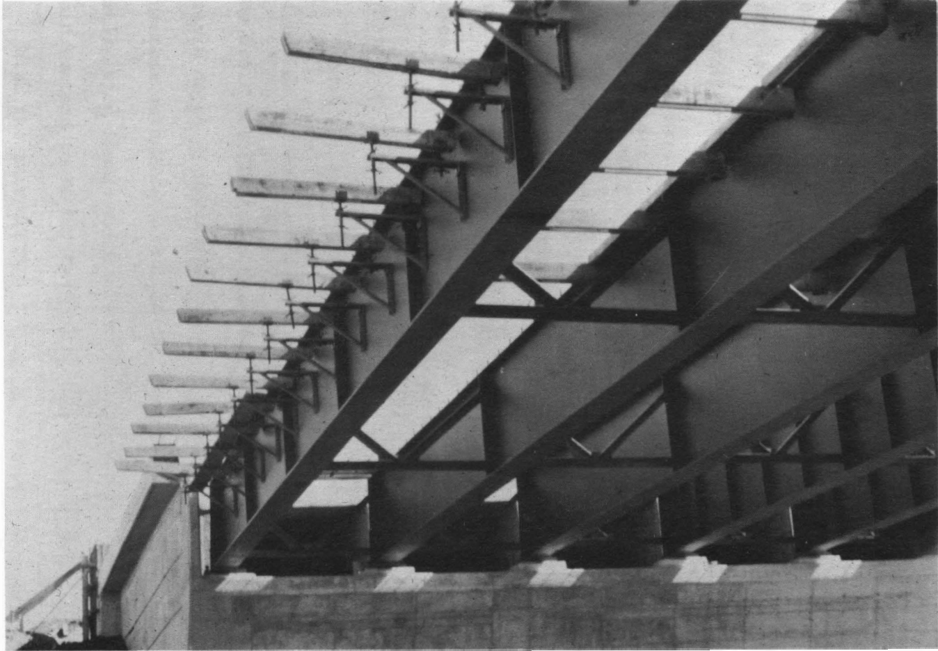
FIGURE 2. Construction Brackets Mounted on Test Bridge Prior to Forming
