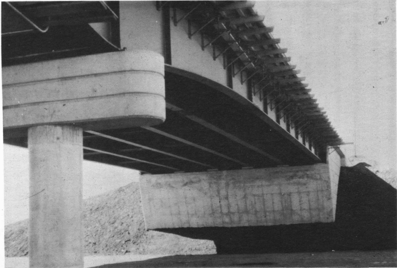
FIGURE 3. Shallow Construction Bracket Mounted on Deep Web
