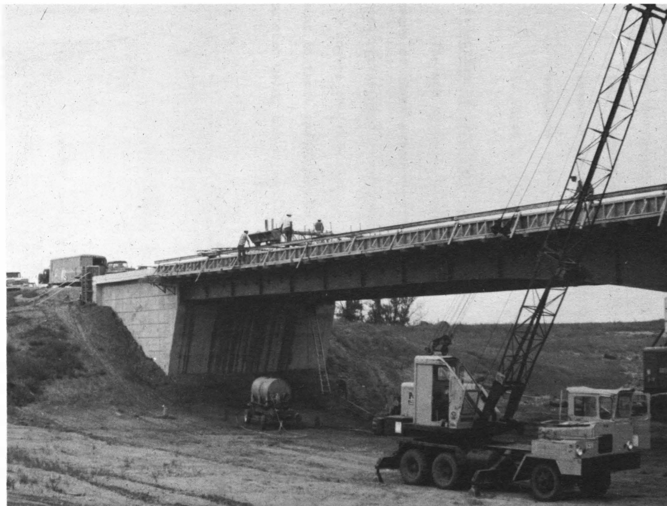
FIGURE 15. General View of Falsework
