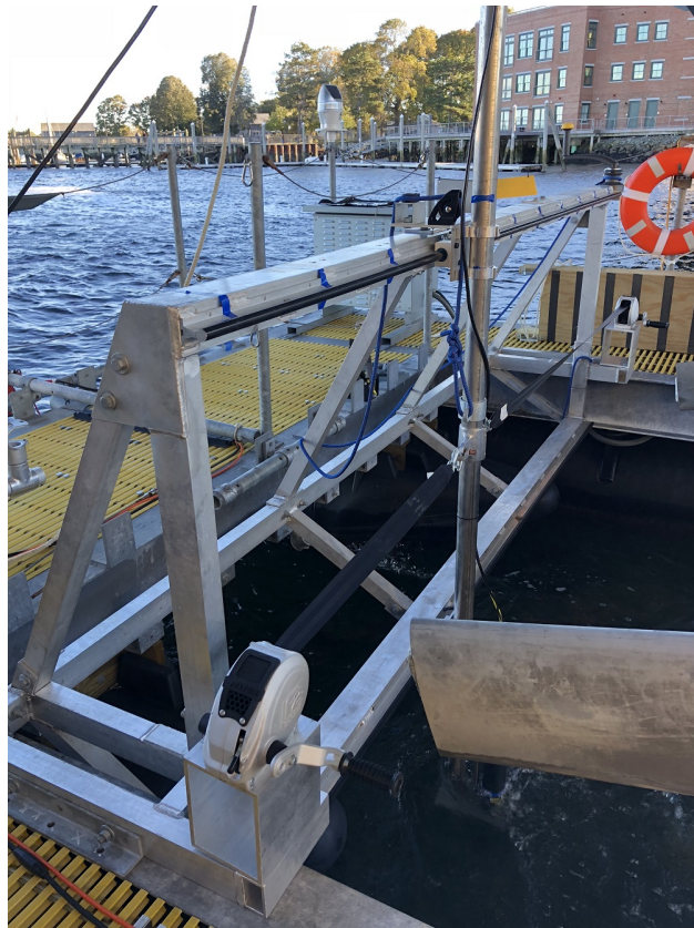
Figure 4.16: ADV traverse installed in the moon pool of the turbine deployment platform
