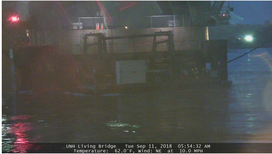
Figure 5.9: Log observed on September 11, 2018 stuck on the platform and bridge pier
