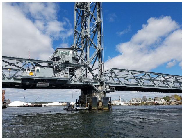
Figure 1.4: Tidal energy conversion system at the Memorial Bridge
