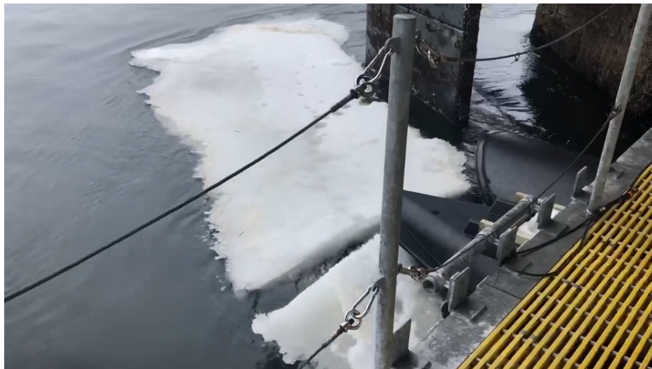
Figure 5.10: Ice chunk observed impacting the turbine deployment platform in March 2019
