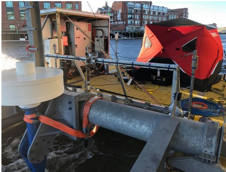
Figure 5.3: Cold weather shelter set up on the turbine deployment platform
