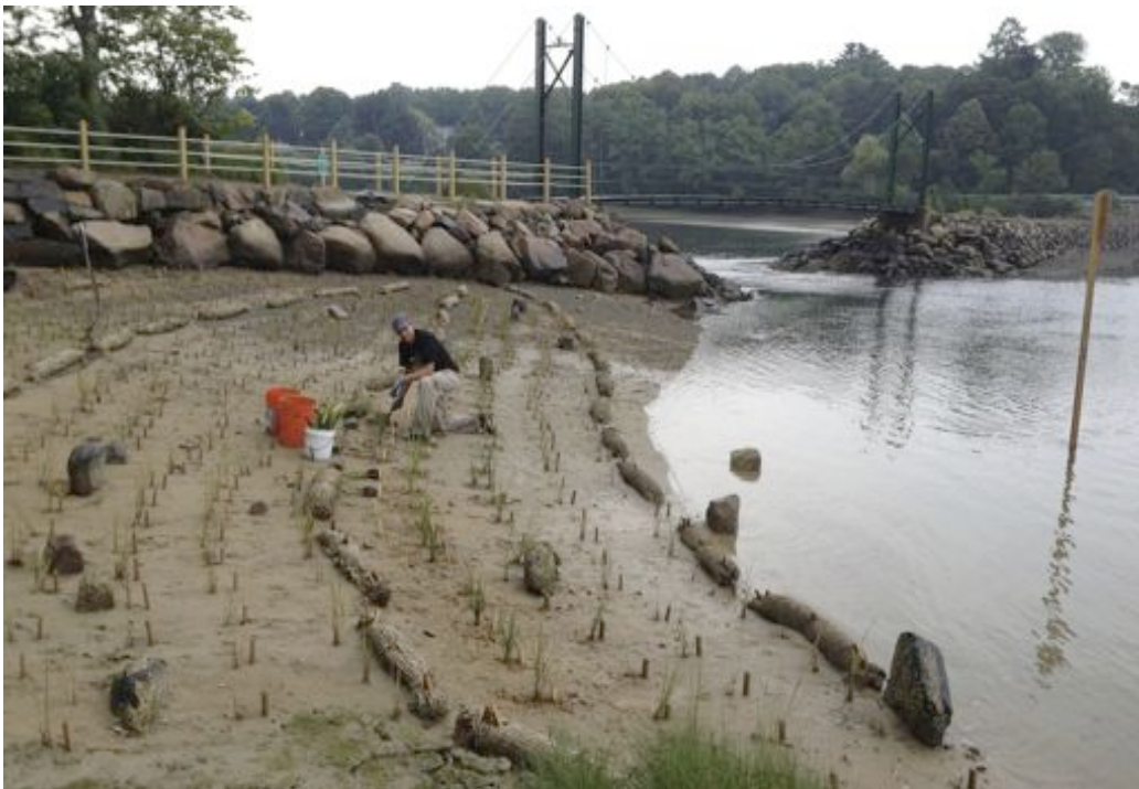
Figure 5. River planting site with biodegradable wave baffles and boulders.
