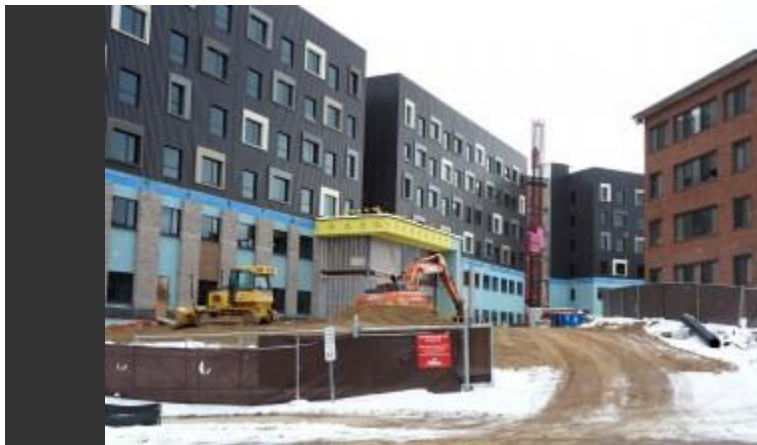
Arcadia Flats will open to students in fall 2020.
