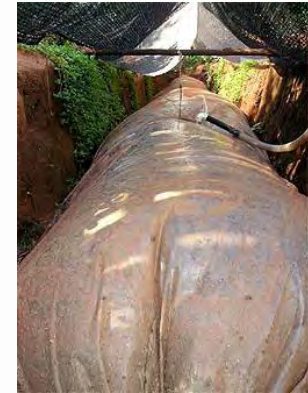
Biodigestor.
