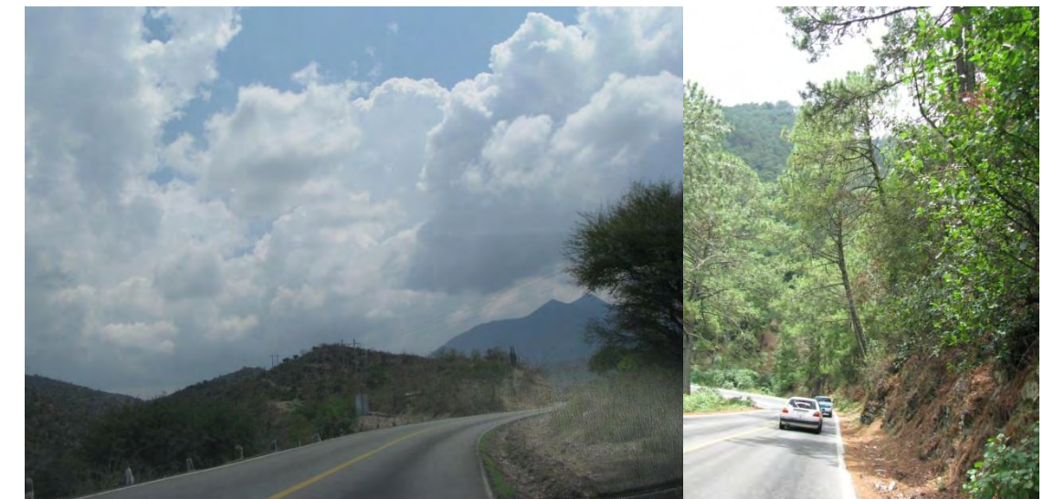
Carretera Federal 85 Zimapán-Tamazunchale
