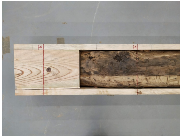
Figure 58 – B-I-NG-1: plank located in the intrados of the beam.
