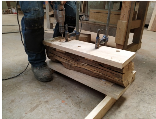
d) Coring of the holes for the pegs.
