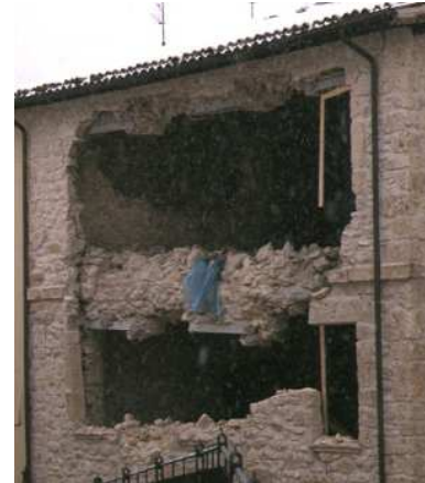
Figure 3 – Example of strengthening with concrete slab after seismic event.[12]
