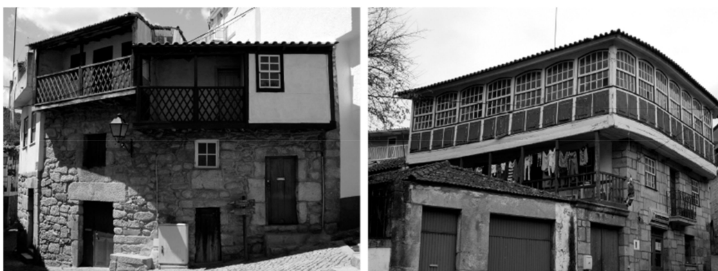
Figure 1. Balconies in the vernacular architecture of Beira Alta, Portugal.
