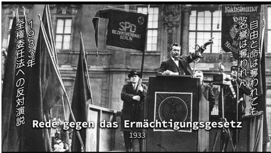
Figure 6. Various semiotic channels transmit information at the same time in Er ist wieder da . The banner of the SPD can be seen at the top of the picture in the middle. Its caption is not rendered in the subtitles, probably because there is not enough space to display all of the information contained in this scene (audio from the dialogue, visual information from the picture, visual information from the on-screen text). To aid the viewer, the term SPD was introduced in a subtitle just before this picture appeared on screen (Fig. 5).
