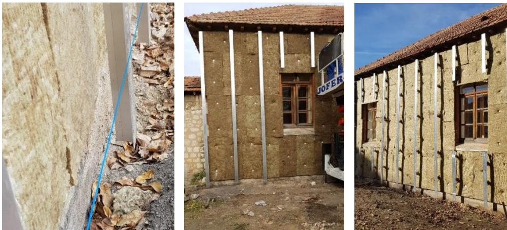
Figure 3. Placement and plumb of the vertical profiles.
