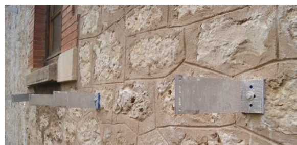
Figure 1. Metal brackets for fixing vertical profiles.
