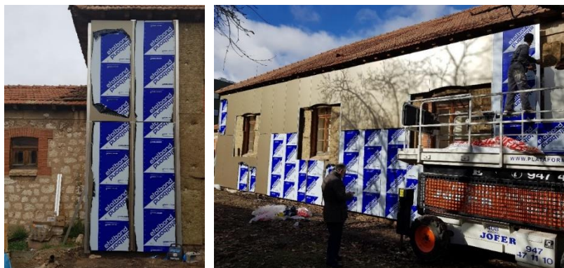
Figure 4. Final cladding placement.
