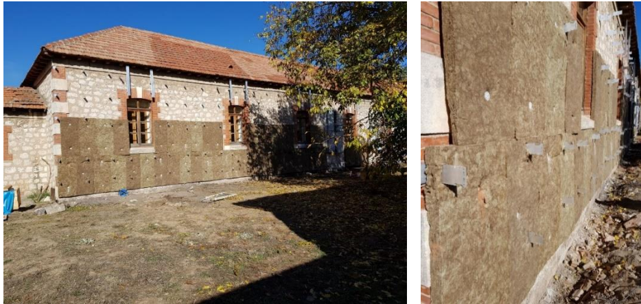
Figure 2. Installation of thermal insulation.
