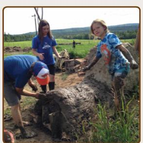
structures letting the layers dry when they reach a certain height to prevent sagging. Continue layering the mud brick until the entire two-part structure is covered. Let dry for a few days.
