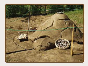
Create a snug door out of a plank of wood to cover the entrance to your newly formed earthen oven. Build a fire in the inside of the oven and stoke with larger
