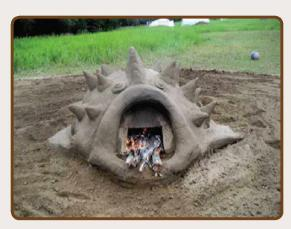
This is an earthen oven in its simplest form. Of course, you can elaborate in all aspects of the building process to create a structure that is more permanent by building a foundation first under the oven, finding a ratio of door size to oven size for better air flow or by making a fancy door to cover the entrance.
