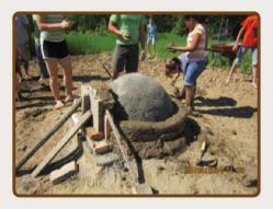
done easily by mixing the sand with water so it will hold its shape. The size can vary depending on what size you want the inside of your oven to be. When the dome is formed, smoothed and packed down, you are ready to start applying mud on the sides and over the top. Have the children make mud "bricks" that are not too wet but are firm, and begin stacking them all around the sand dome. First make a
