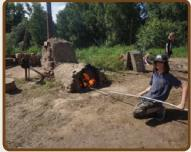
When dry, cut an arched door in front of the fire chamber to use as the entrance for placing wood into the fire chamber. Cut another arching door into the side of the pottery holding chamber. This entrance will be used to place the pottery inside the kiln when ready to be fired. After the pottery is placed inside this entrance it will be bricked and mudded over to cover the entrance so all the heat
