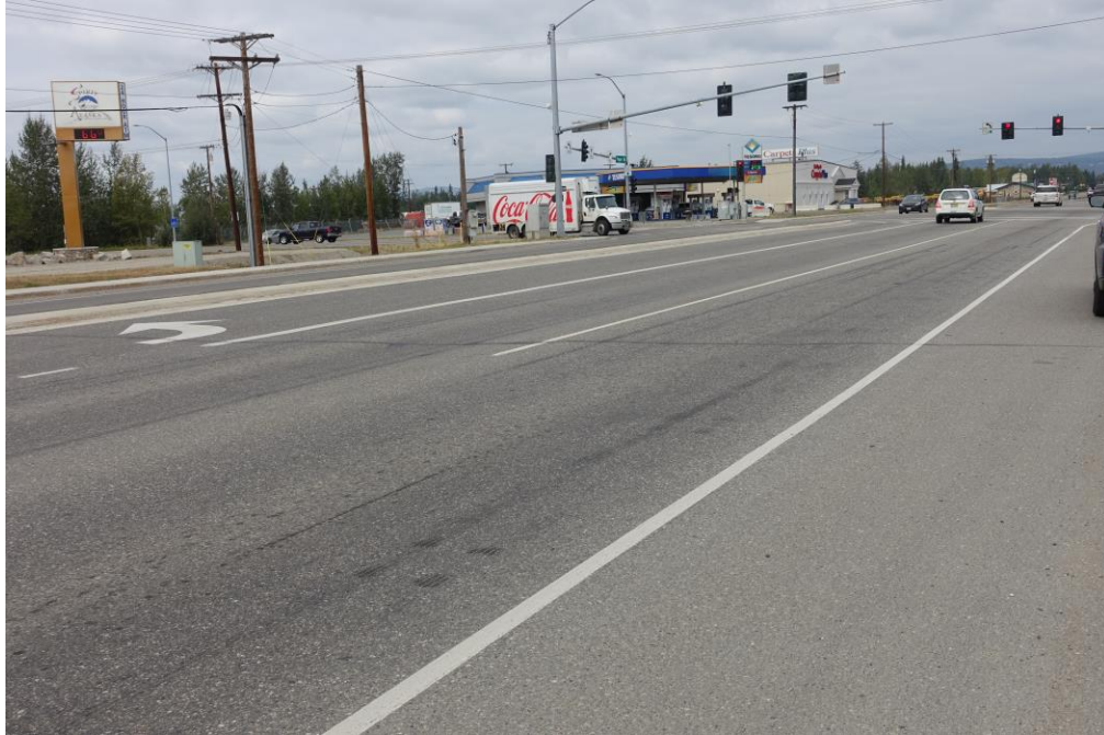
Figure 4.54 Peger Rd Resurfacing / FMATS Ped Impr / NR Signal Interconnect, PG 52-40, constructed in 2017
