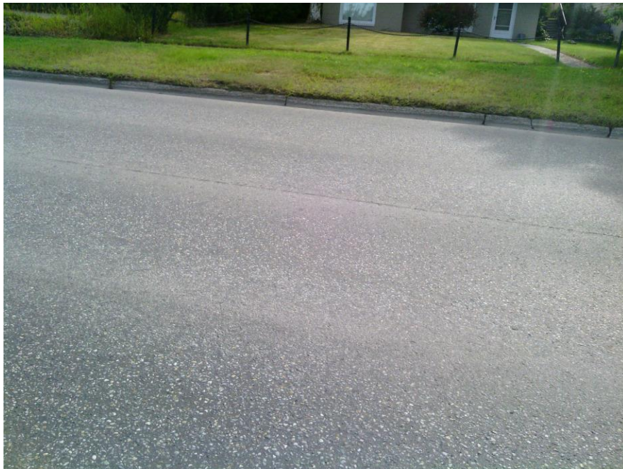
Figure 4.55 L & I Couplet and 5th & 6th Avenue Couplet, PG64-40, constructed in 2014/2015
