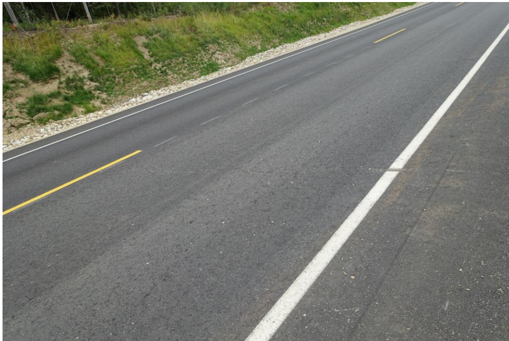
Figure 4.53 Old Nenana/Ester Hill Rehabilitation, PG 52-40, constructed in 2018
