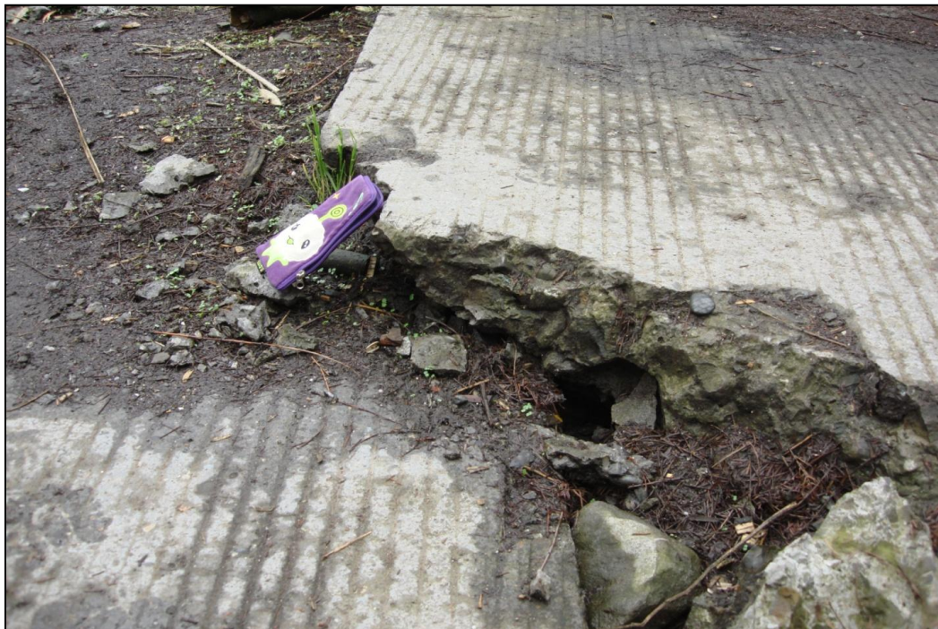
Figure 2.5: An example of the 'slip' along the fault line
