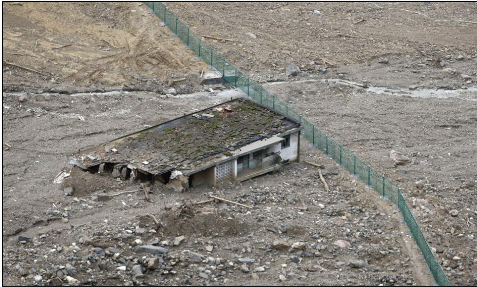
Figure 7.41: Chain-link fencing may be seen everywhere in Beichuan
