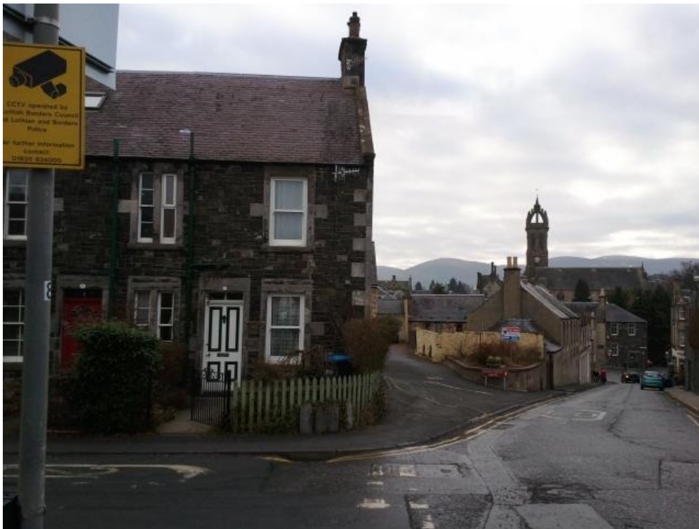
Figure 39: Julian Goodacre's home (left) and workshop (the building down the hill to the right, behind the red, white, and blue sign) in Peebles, Scotland.
