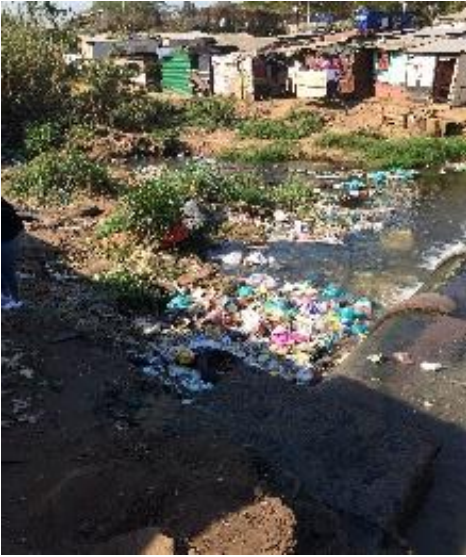
Strom water channel in Quarry road flooded with refuse
