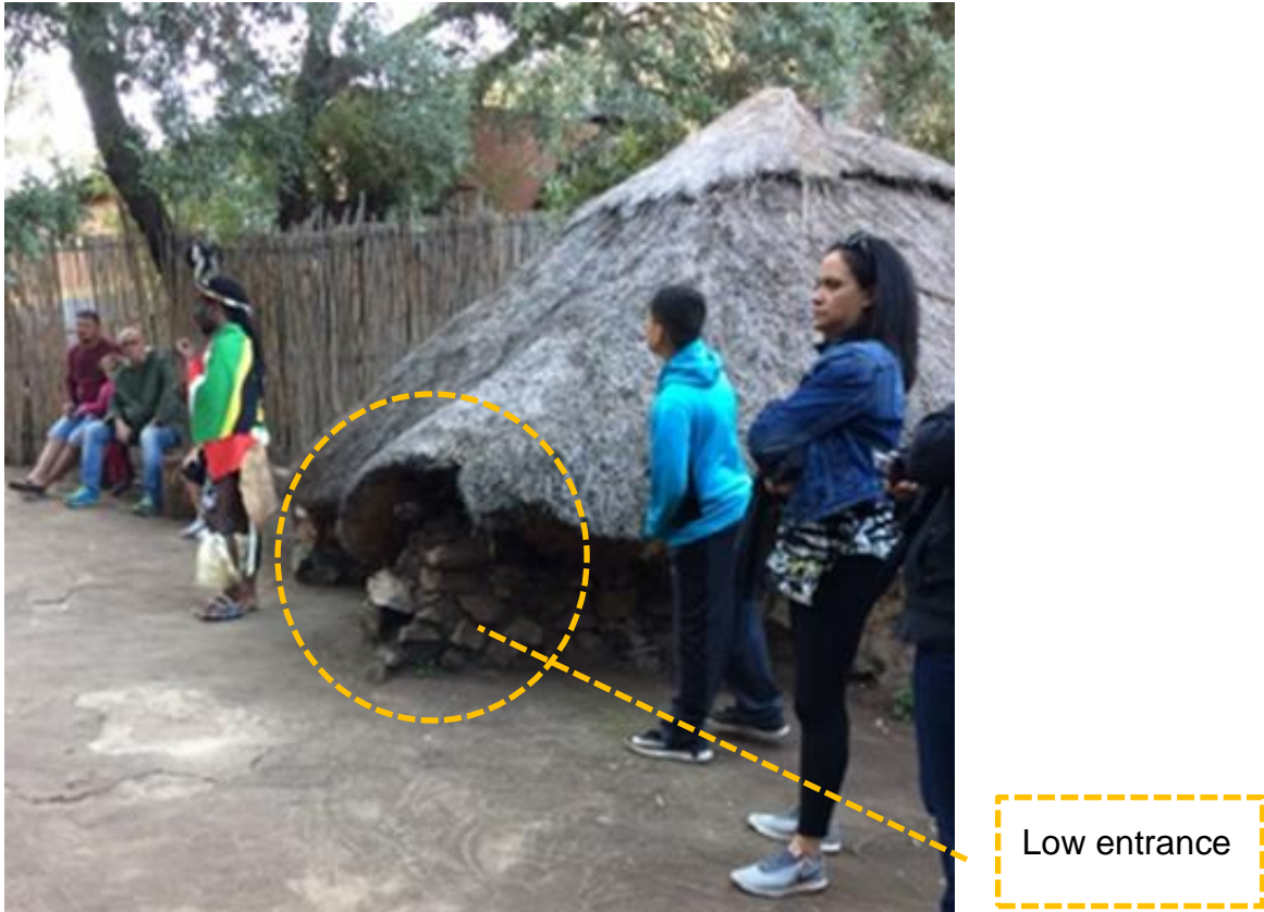
FIGURE 4-2 TRADITIONAL HUT WITH LOW ENTRANCE
