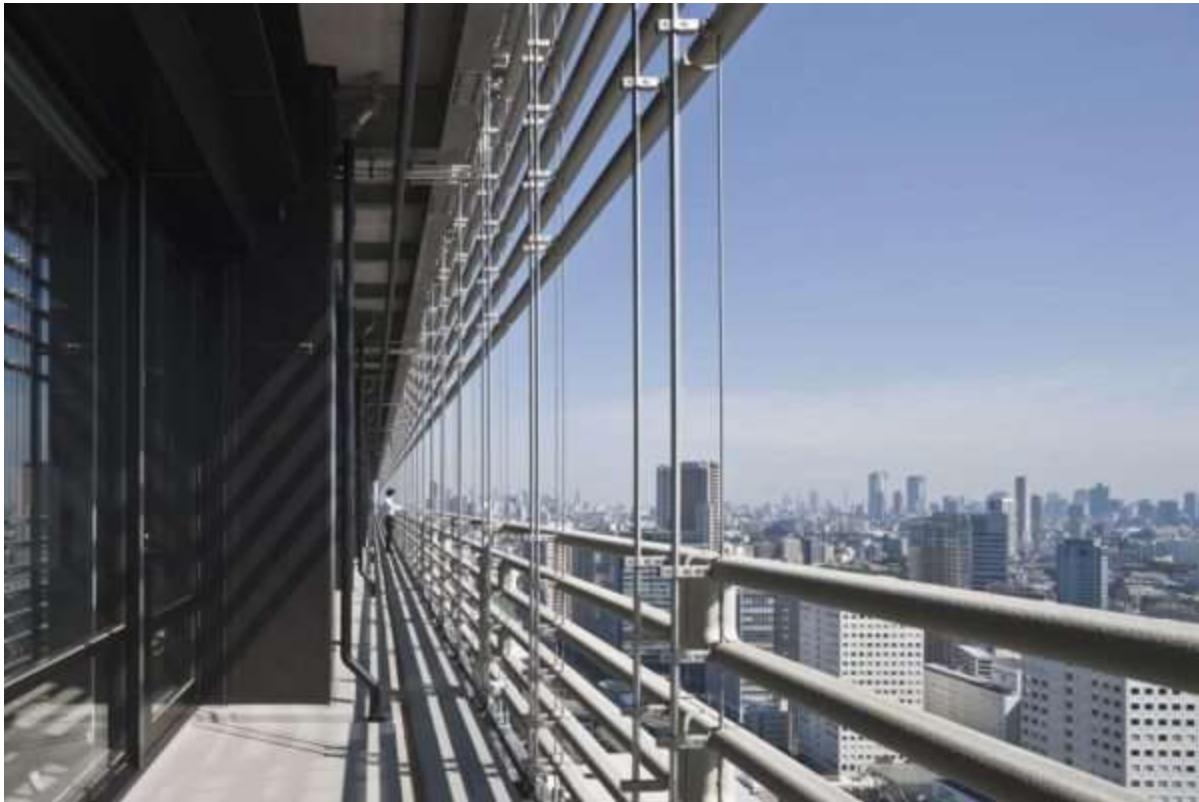
Figure 29: Sony City Osaki Building utilizes a BioSkin to cool the surrounding air. Source: materialdistrict.com, 2016
