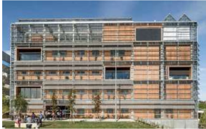
Figure 5: The new headquarters of the Institute of Environmental Science and Technology and the Institut Català de Paleontologia (ICTA-ICP) in Barcelona is wrapped in a responsive, bioclimatic skin which reduces water consumption up to 90% and energy consumption levels by 62% Source: Inhabitat, 2015.
