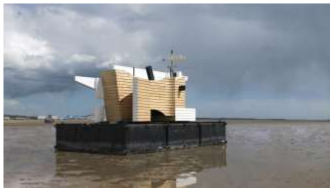
Figure 4: Flood house adapts to its immediate environment, rising and falling with the tides of the Thames estuary. Source: Brotherton Lock, 2016
