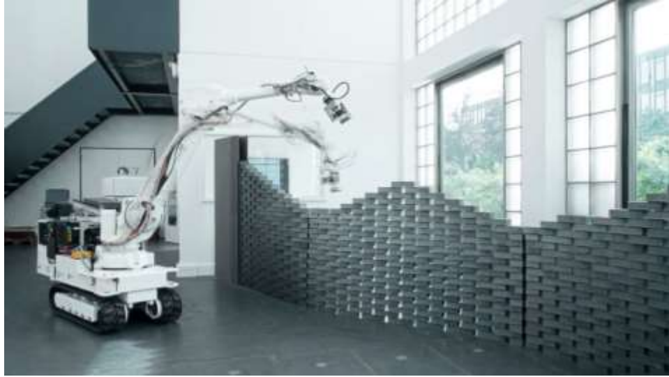
Figure 23: In-situ fabricator, NCCR Digital Fabrication. Source: robohub.org, 2015
