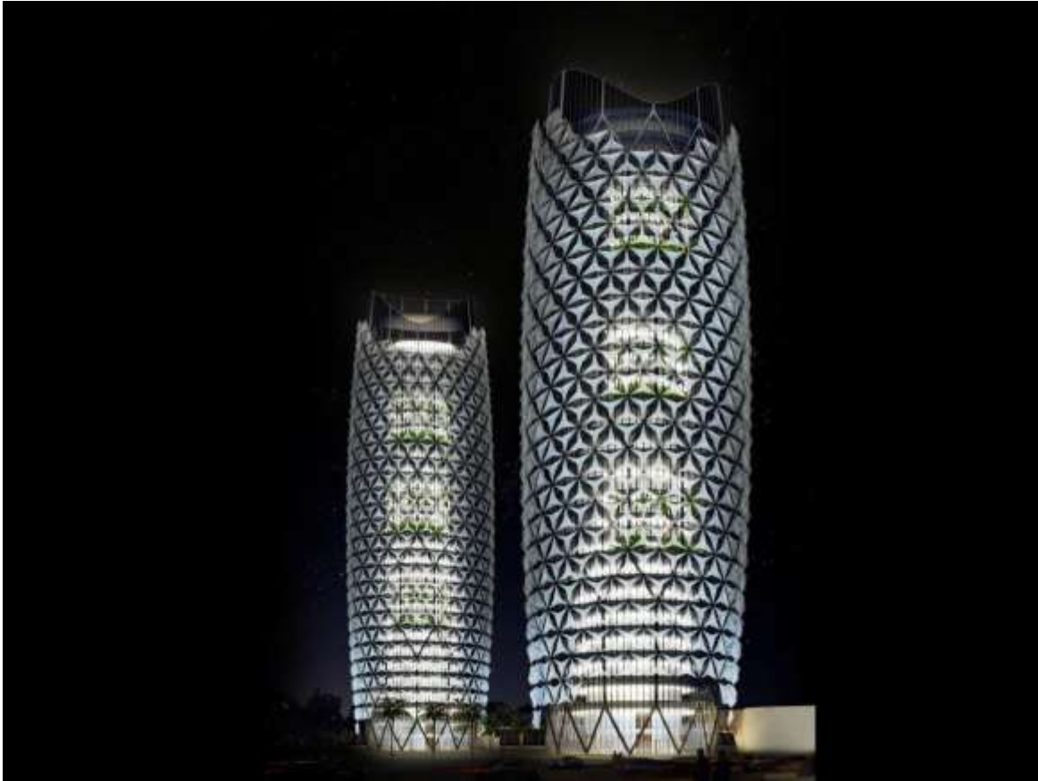
Figure 62: Aesthetically, the façades expression is firmly rooted in the rich cultural context of the UAE. Source: archdaily.com, 2012
