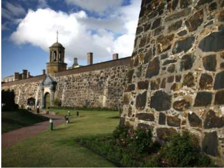
Figure 73: Cape Town Castle or the Castle of Good Hope was constructed in 1666 using Malmesbury Slate. Source: www.portfoliocollection.com/visit/castle-of-good-hope-and-iziko-william-fehr-collection , 2015
