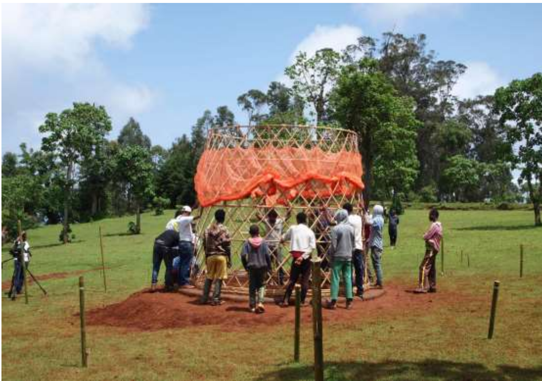
Figure 49: Warka Water Towers are designed in such a way as to let the local communities learn how to build it themselves and replicate it as needed. Source: www.dezeen.com , 2016
