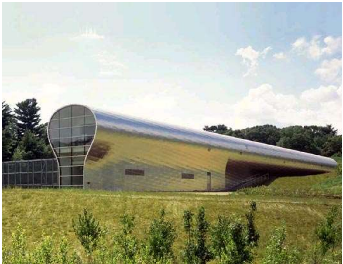
Figure 55: The 12-metre-long sliver takes its form from a water droplet. The steel shingles which clad the building reflect the environment whilst simultaneously dissipating any heat gain through the edges. Source: http://www.stevenholl.com , 2007
