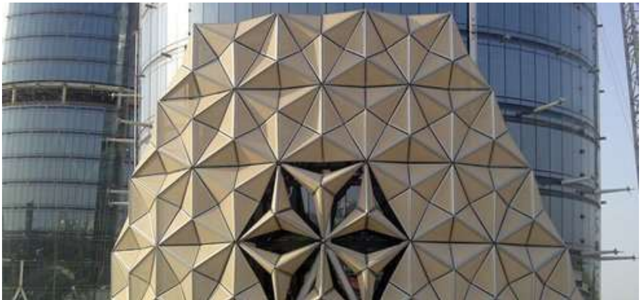
Figure 59: Inspired by traditional Islamic shading devices, this kinetic facade responds to the movement of the sun to control the solar gain in the buildings. Source: https://www.archdaily.com , 2012
