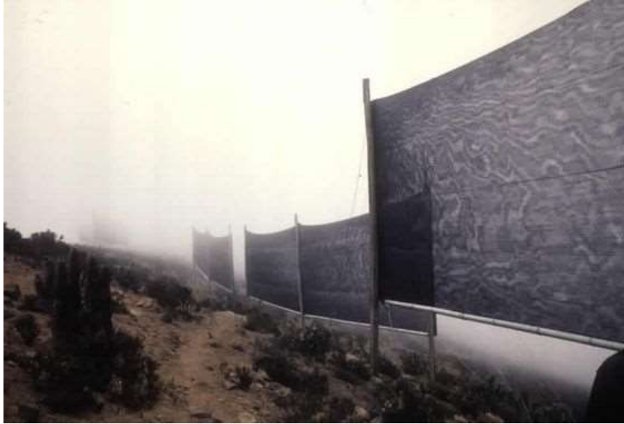
Figure 33: Standard fog collectors in the Atacama Desert, Chile, consisting of Raschel nets spanned between two upright posts and a horizontal gutter, and anchored with cables. Source: quemaoviejo.com
