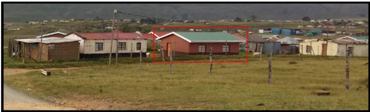
Plate 5.6: Single-detached Housing Structures provided in situ
