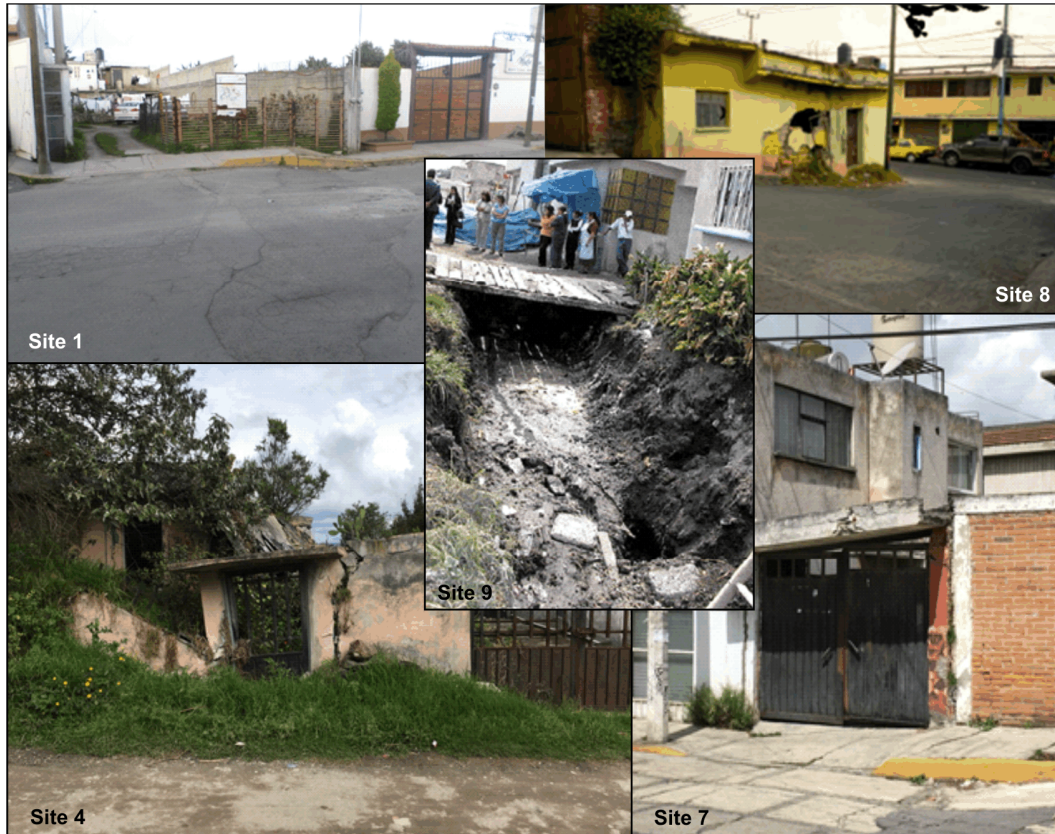
Figure 13. Examples of ground fractures observed in the field while surveying the areas identified by PSI. The locations visited are all marked on Fig. 12.
