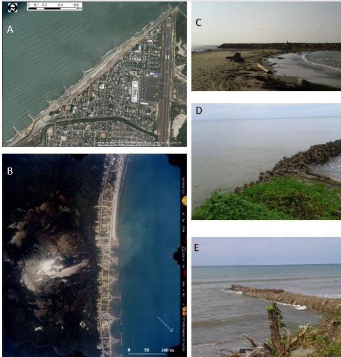
Figure 1.11. Shore protection structures in the Caribbean littoral. Upper Sector of Marbella in Cartagena city (Bolívar), where a battery of groins is trapping sediments from the longshore drift towards the southwest (source: Esri Imagery); Down: Southern part of the Gulf of Morrosquillo (Sucre), where a sequence of breakwaters and T-shape groins that do not succeed in stabilizing the highly intervened sandy barrier in front of extensive mangrove swamps. Courtesy of Eafit University.
