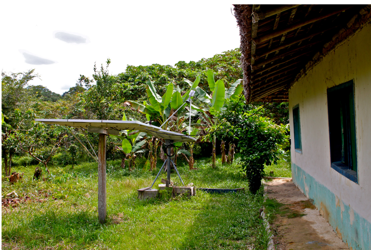
Gesac Antenna and solar panels at Pamáali School
