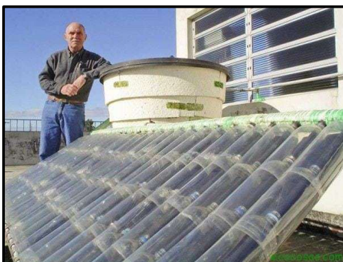
Image 7. Solar water heater
