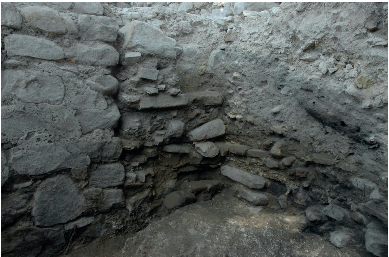
4. Piso (C8) de acesso à primeira torre circular da cerca a Sudoeste do castelo, em 2016. Pavement (C8) giving access to the first round tower of the urban wall to the southwest of the castle, in 2016.
