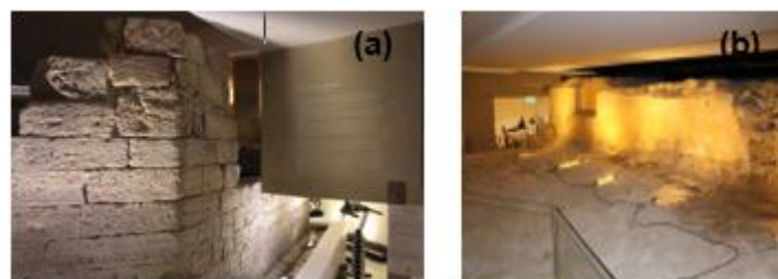
Figure 8 – Corpo Santo Hotel: (a) João Bretão Tower and (b) nucleus of the tower
