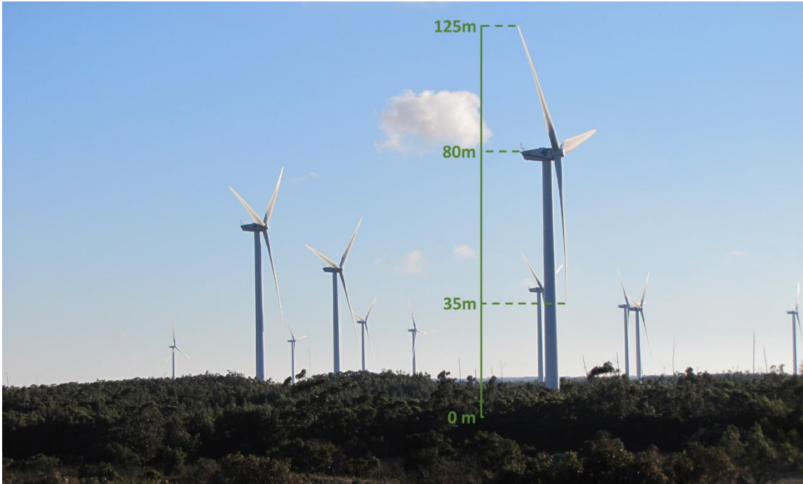
Figure 3: Turbines at the BSJWF, showing the nacelle height and minimum and maximum heights reached by the blades.
