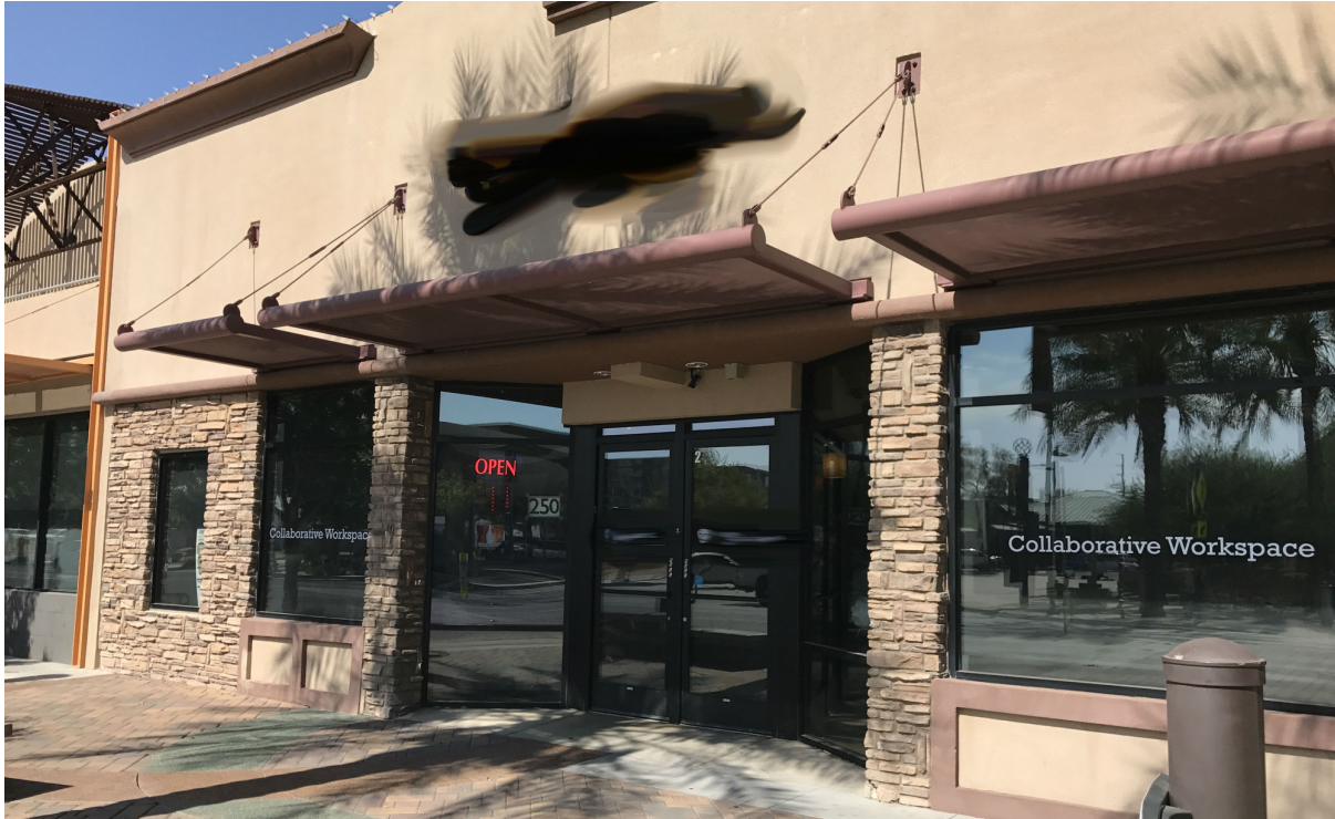
Figure 2. Close-up view of the front entrance of Technology HQ.
