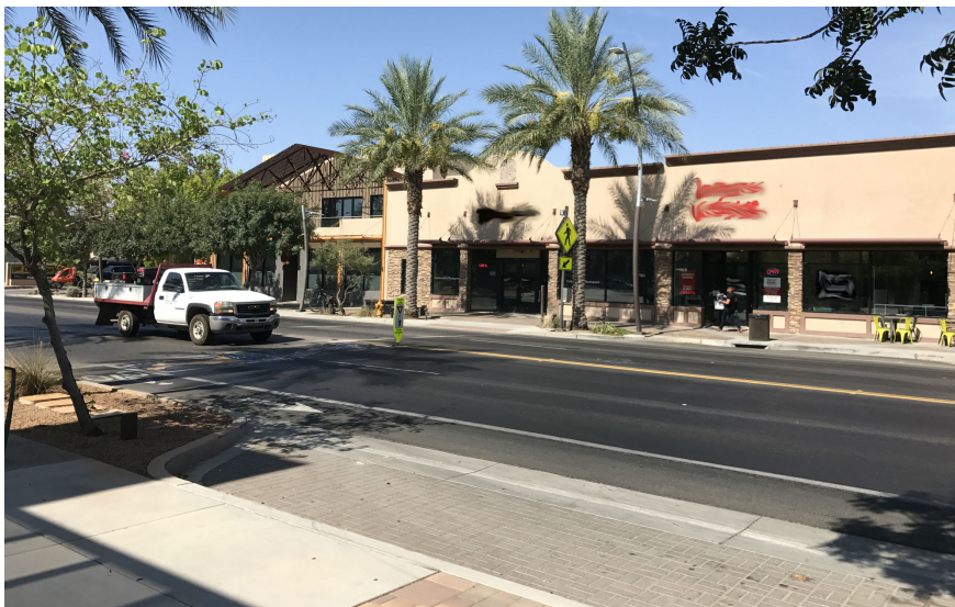
Figure 1. Exterior view of Technology HQ (left) occupying half of a commercial center on a major street in a Phoenix, AZ suburb.
