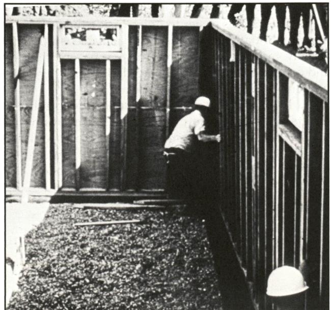
Figure 2. Plywood sheathing covers the PWF.
