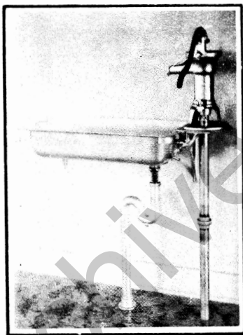
Fig. 1.—Pump, Sink and Drain—A convenient low cost method of bringing water into the kitchen from a near-by cistern or shallow well. The sink with drain makes easy the disposal of most of the kitchen waste.
