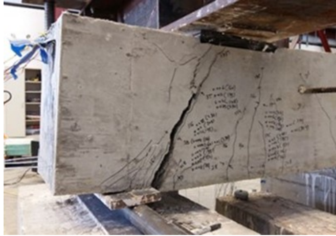
Figure 3.7 Pullout failure – Specimen H-3-8-5-11-F4.1-2
