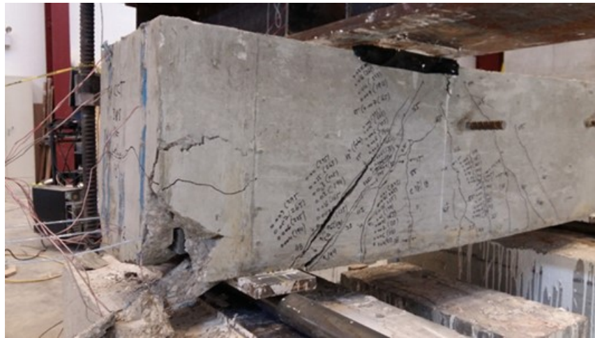
Figure 3.2 Specimen H-3-8-5-13-F4.1-2 after failure
