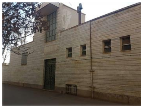
Figure 1. Real building in Isfahan city.
