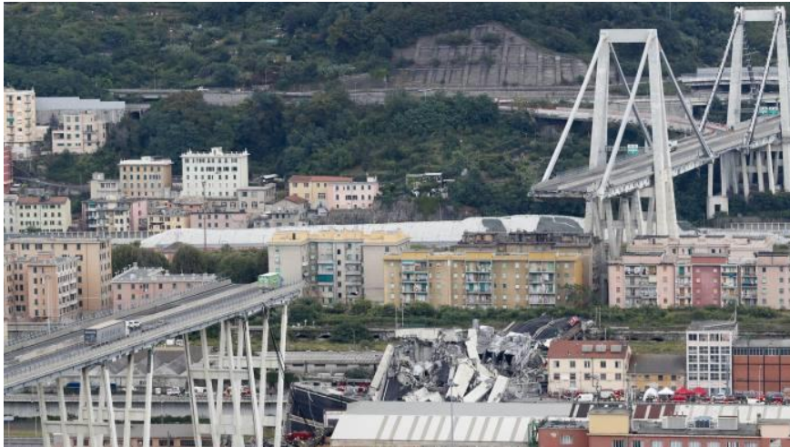
Fig. 1.1 The collapse of Morandi road bridge in Genoa.
