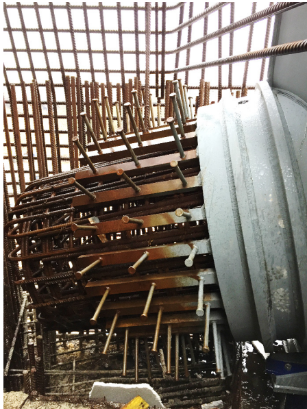
Figure 2. Arch spring connectors.
