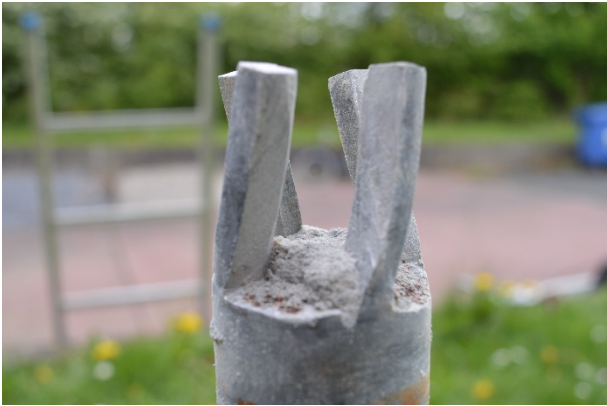
Figure 7. Excessive bending of strips.
