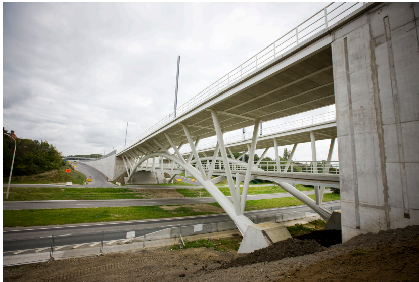
Figure 1. Overview of Woluwe Lane Bridge.
