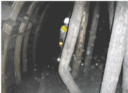
Figure 3. The fragment of a state of the zonal mine working support with a decreased rigidity of the collapsed rocks in the mined-out space
