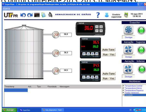
Fig. 5. Supervisory software screen. The software collects and saves all of the data generated by the electrical control panel during the control of temperature.
