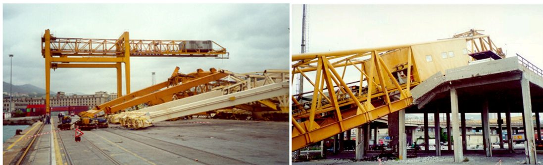
Fig. 2. Consequences of the downburst occurred in the Port of Genoa on 31 August 1994.
