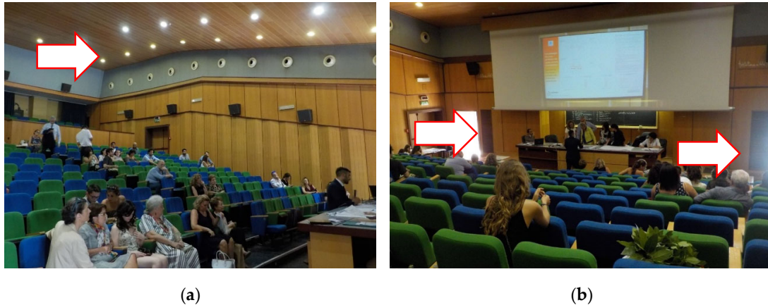
Figure 4. Top view of Aula Magna (a) High induction diffusers; and, (b) Air extraction vents.
