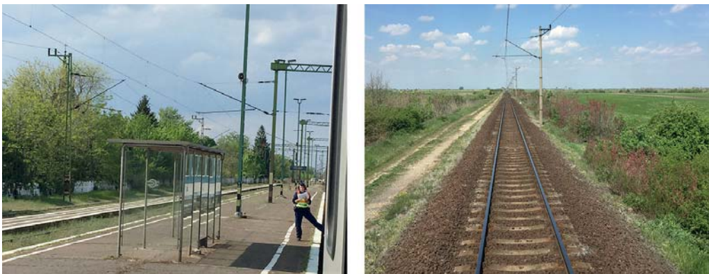
Fig. 2: Corridor capacity and performance challenges Budapest–Beograd: waiting times at borders (e.g. Kelebia, Hungary, left) and single-track infrastructure produce travel time losses / Source: Author
