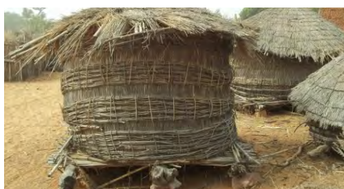
Photo 42: A poorly built storage structure
