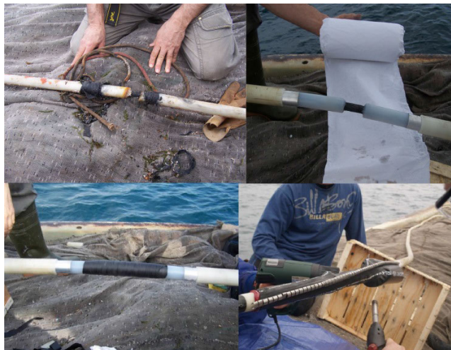
FIGURE 13. The cable before and after the repairs.
