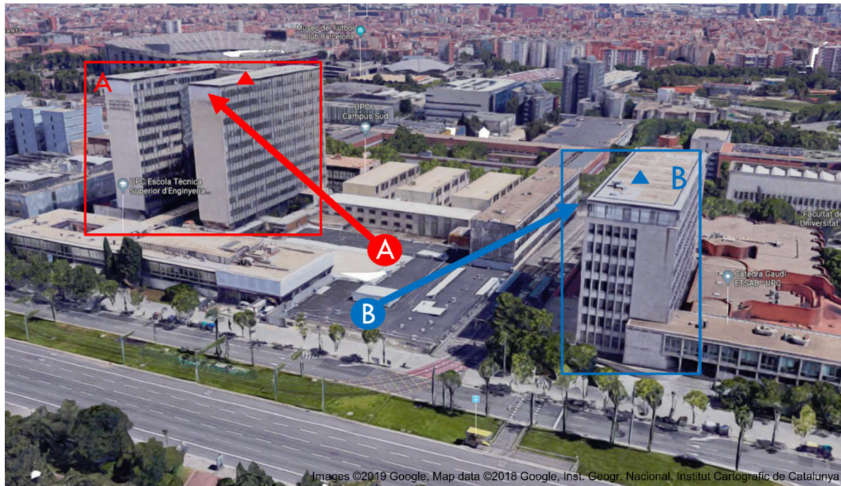
Figure 2: Building A (left) and building B (right), the circles indicate the sites where the RAR device was located and arrows correspond to the LOS. Triangles show where the accelerometers were placed.
