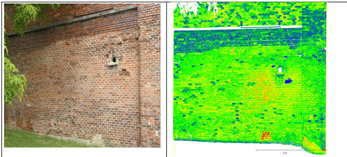
Figure 2. Tested historic brickwork (left) and point clouds of this wall
