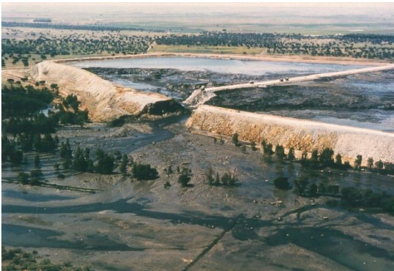
Figure 25. View of Aznalcóllar dam after failure
