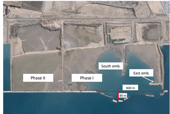
Figure 33. Length of the Prat quay failure and maximum distance travelled by the caissons
