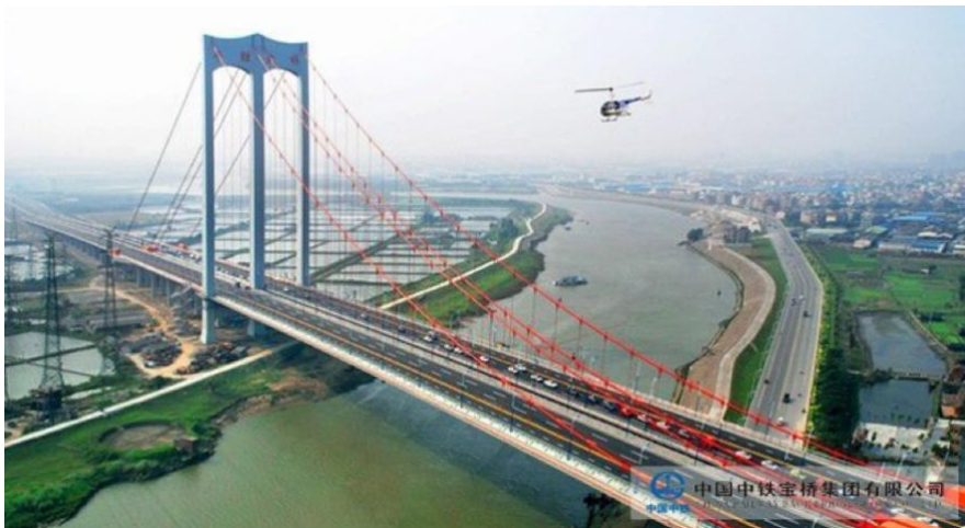
Figure 2.43 Pingsheng Bridge in Guangdong.
