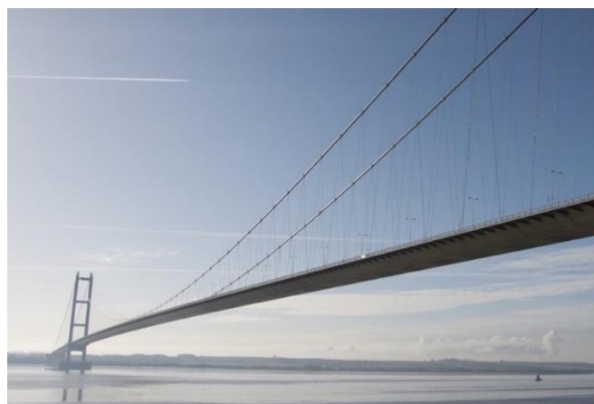
Figure 2.47 Humber bridge, Kingston upon Hull, England, UK.
