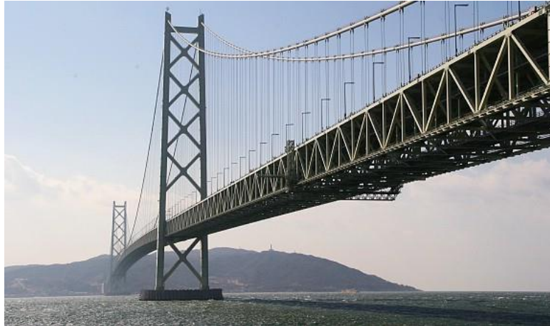
Figure 2.52 Akashi Kaikyo Bridge, Japan.
