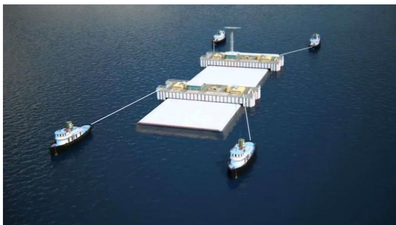
Figure 2.34 SFT elements being towed to the site.
