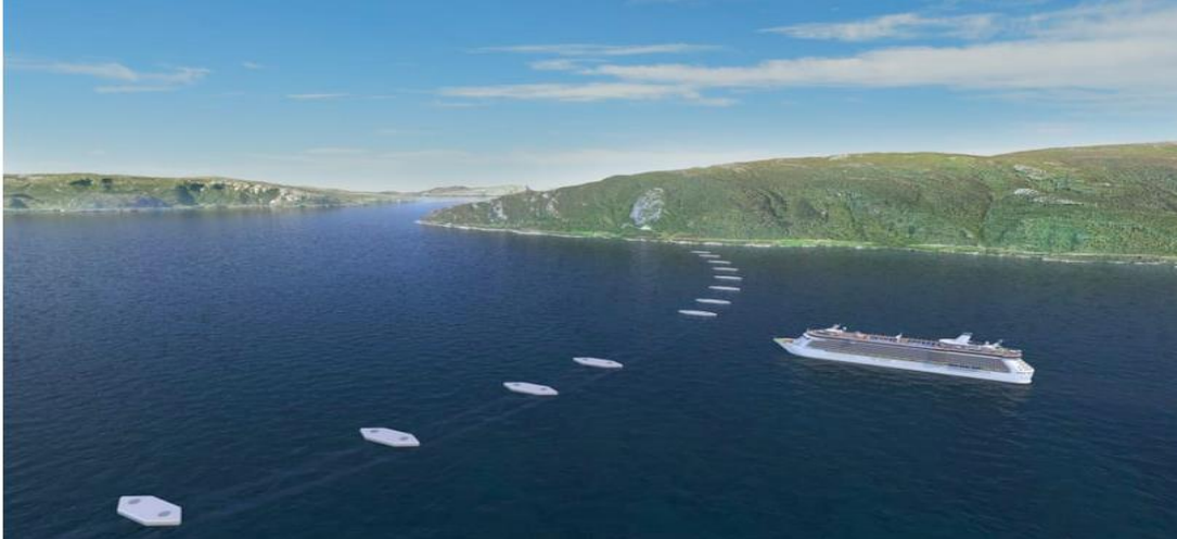
Figure 2.16 A proposed SFT supported by pontoons for the crossing between the cities of Kristiansand and Trondheim.
