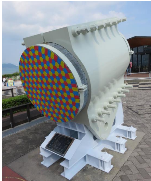
Figure 2.55 Cross section of the main cable in Akashi Kaikyo Bridge (De Miranda M., 2017).
