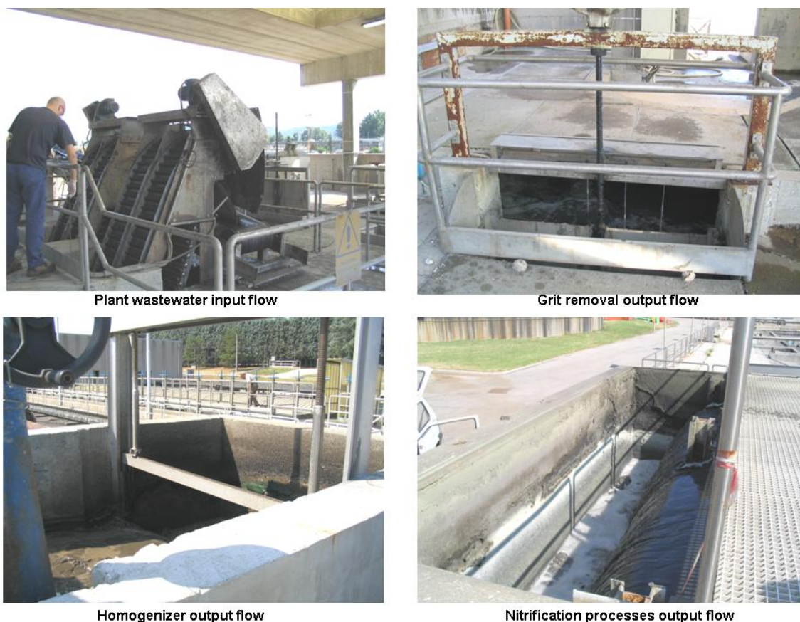
Fig. 5.3.3: the four sites of wastewater industrial line inside the plant, where the samples for the e-nose measurements have been collected.
