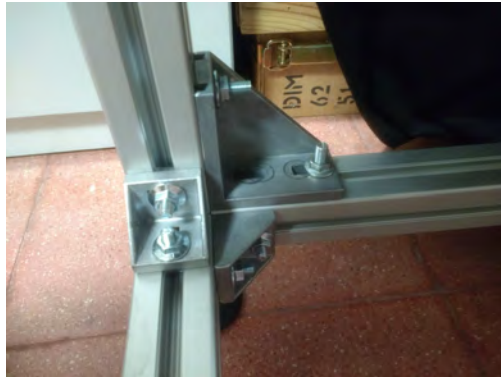
Figure 2.35: Mounted set of brackets and profiles.
