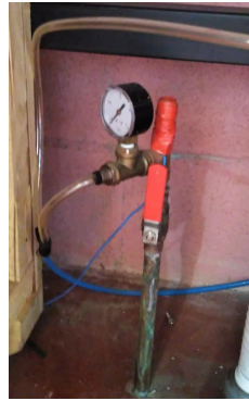
Figure 4.10. UC3M PEMFC laboratory air intake
